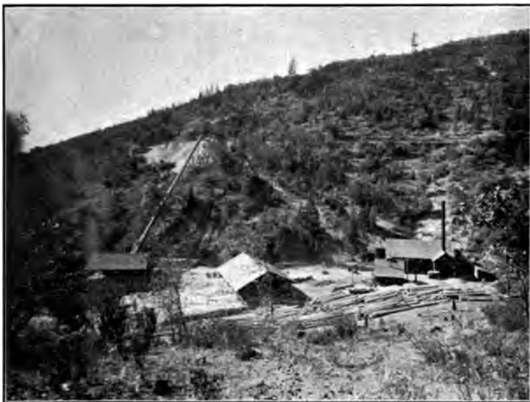
CHUTE BETWEEN TUNNELS Nos. 2 AND 3. ELECTRIC POWER HOUSE, AND TIMBER SHEDS. BULLY HILL MINES.
